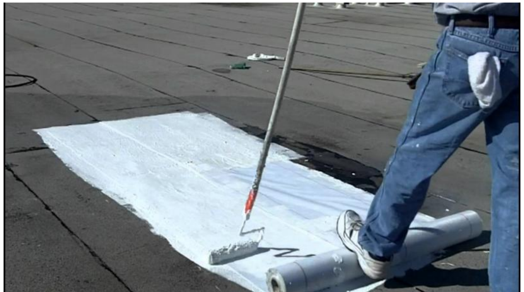
Application of a roll-on liquid applied system over an existing modified bitumen roof. When is a coating not just a coating? When it has separate reinforcing layers included as part of the assembly.
